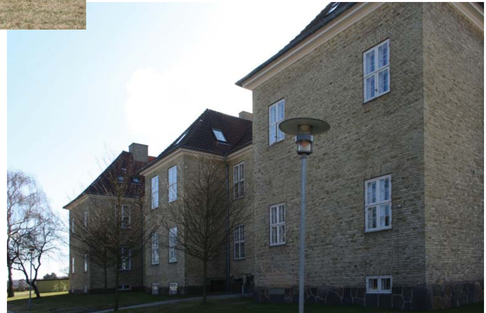
Poppelhus, facade mod nord
