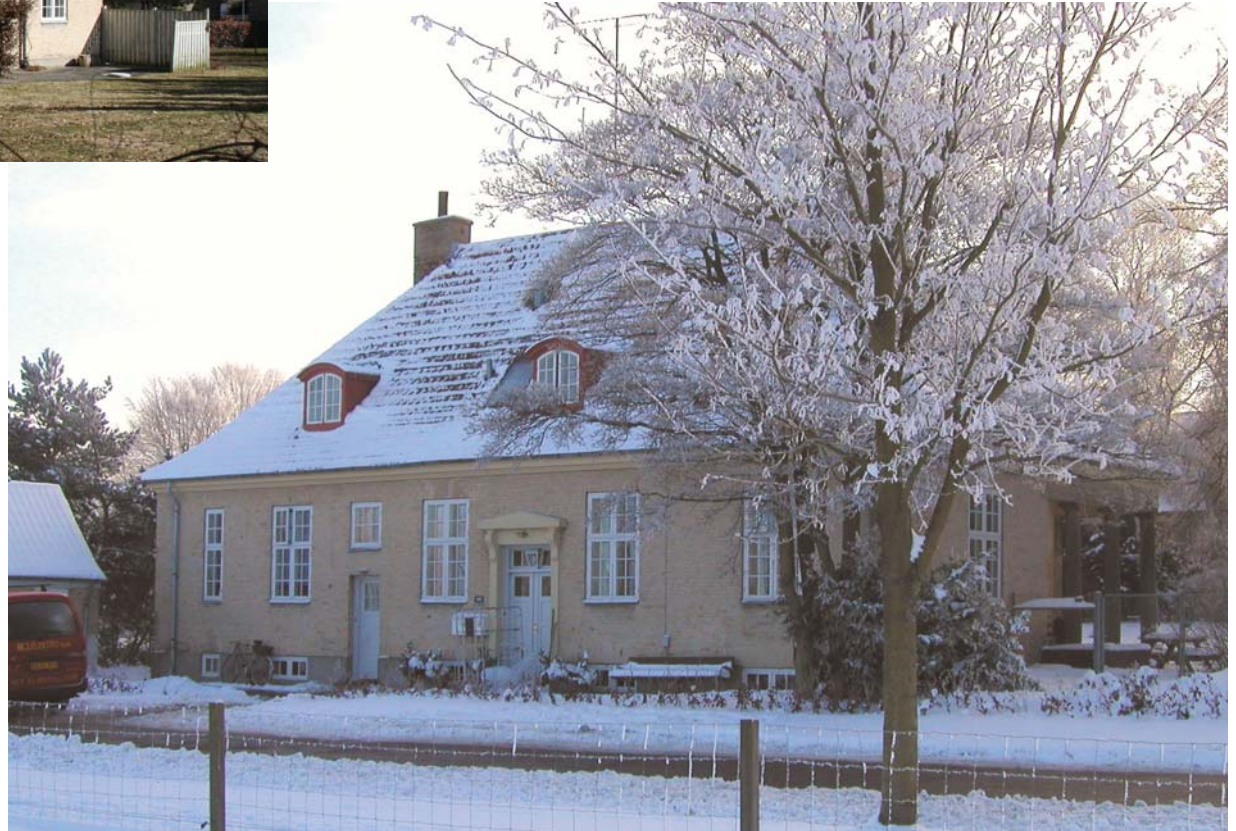
Toftebakken 10, facade mod nord
