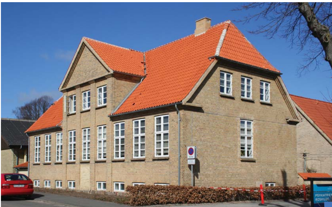
Sct. Jørgensbjerg Skole, facade mod Smedegade
