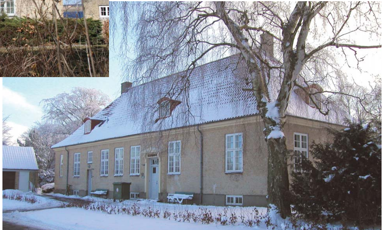
Toftebakken 11, facade mod nord
