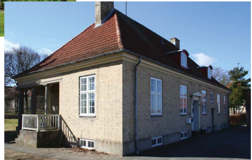
Toftebakken 9, facade mod nord
